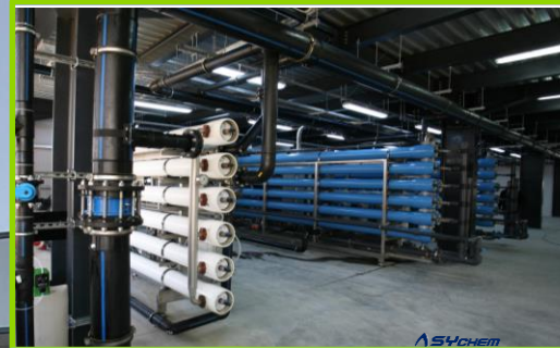
Water Treatment Sector
