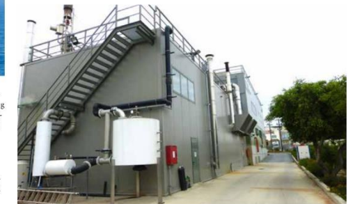
The Heraklion Biogas Plant features here in this part of the facility a special deodorization system that enables plant's integration into the urban environment and a highly specialized wastewater treatment system for the effluents avoiding any contamination of the environment.
